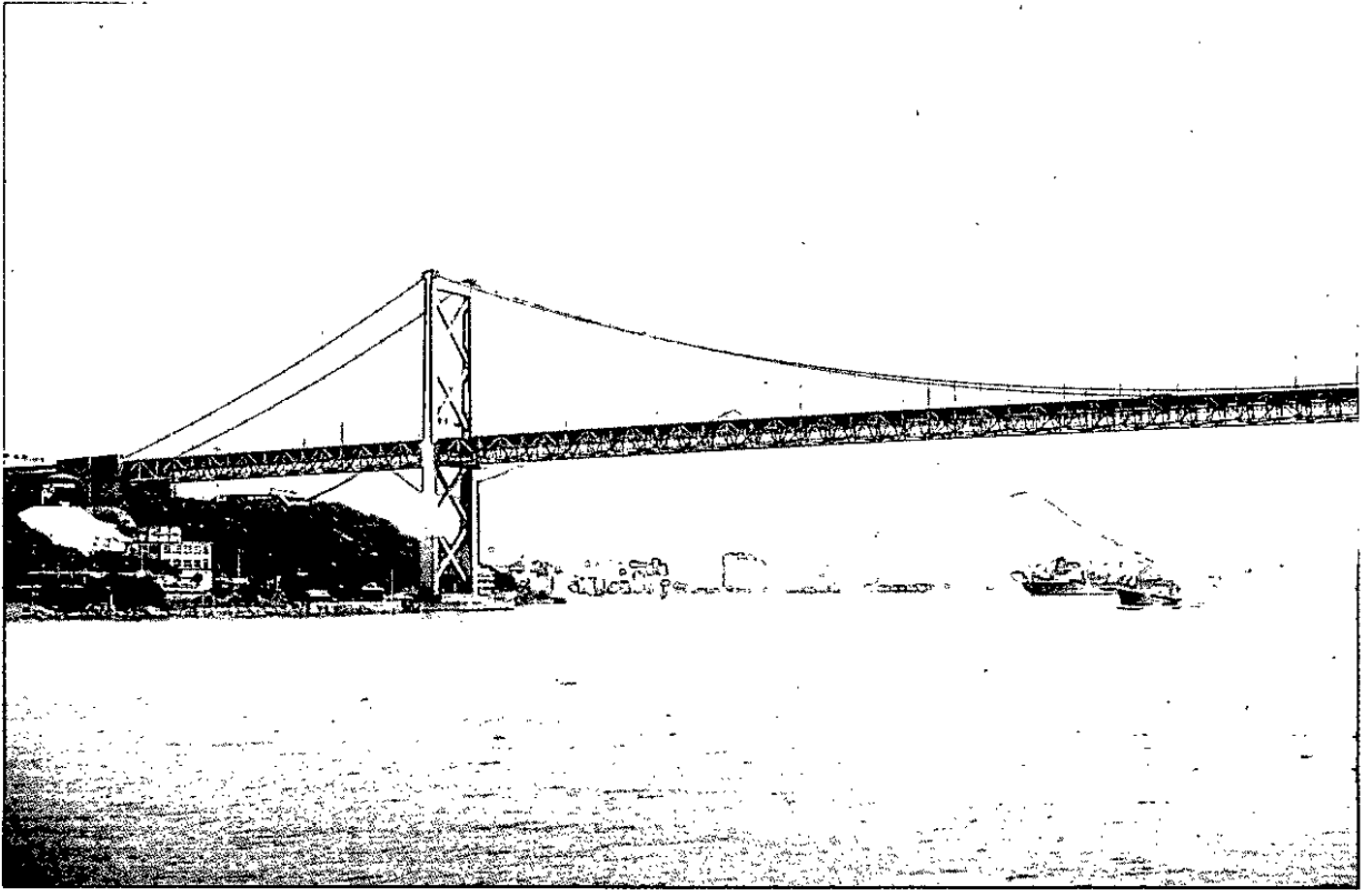
Figure 20: THE KANMON BRIDGE
