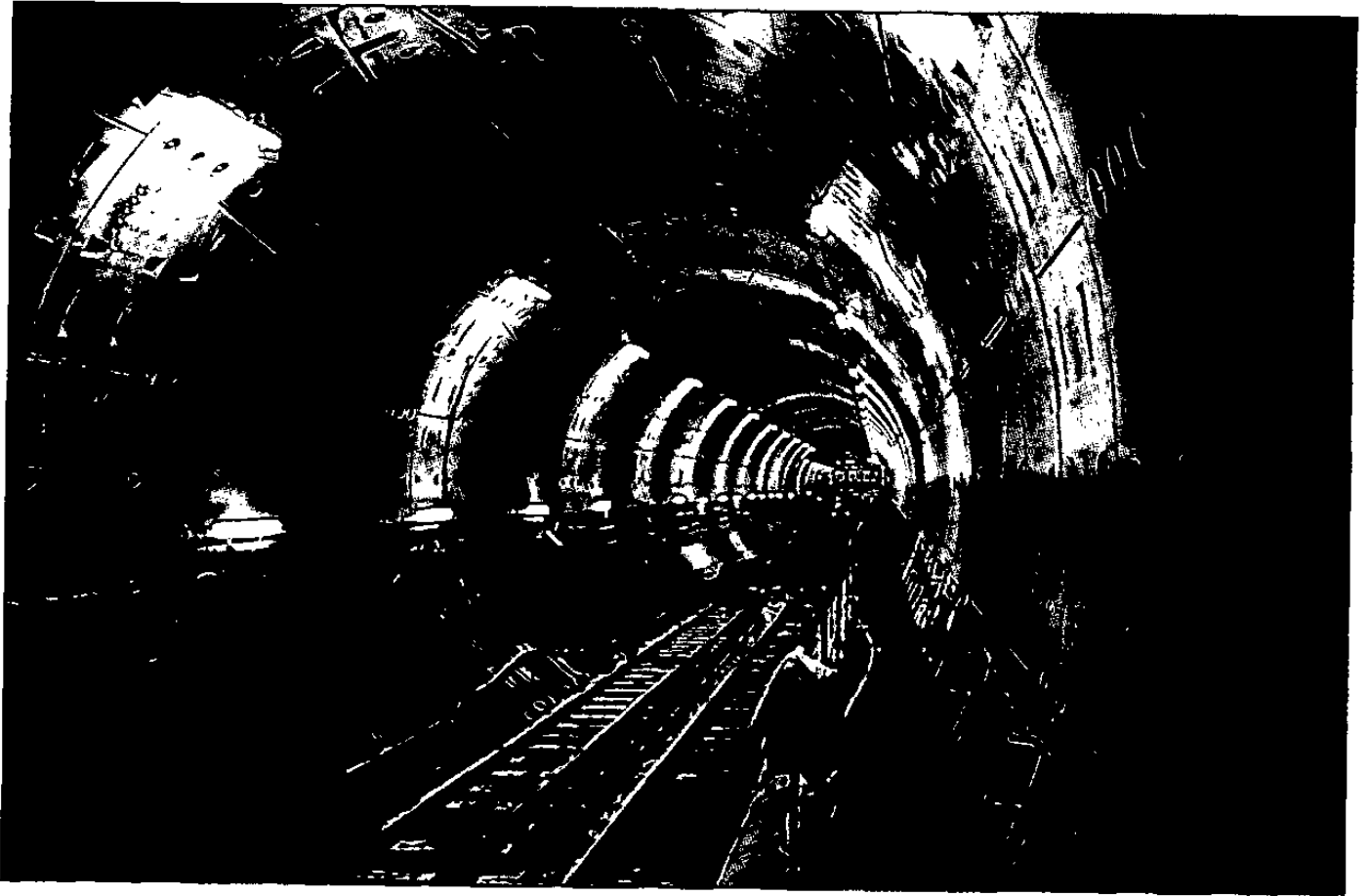
Figure 2: THE EASTERN RAIL TUNNEL
